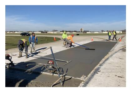
The Airport Authority completed Phase I of a project to remove and replace several airfield concrete pavement panels, isolated drainage structures and hangar apron areas. Total project cost \$435,815.
