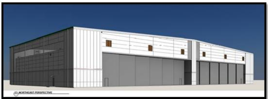
CH2M, the Airport Authority's engineering consultant prepared bridging document plans and specifications for solicitation of a design-builder to construct a 48,000 SF, two (2) bay tenant hangar to be constructed on the South High Tail Ramp in 2022/23.
