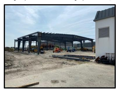
The Airport Authority is constructing a 16,500 square foot expansion on the east side of its existing maintenance building. The new expansion will accommodate the existing fleet of equipment and materials utilized by Airport maintenance departments.
