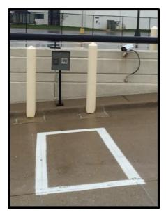
The Airport Authority replaced its access control system hardware and software, which was more than 10 years old. The replacement included 54 access card readers at gates along the eight miles of perimeter fencing in addition to servers, network communications equipment, and existing software platform.
