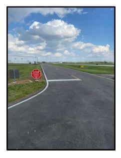
Under the Airport Improvement Program (AIP) Federal and State grant funding, the Airport Authority constructed a roadway that connects pavement at the Echo 1 Hangar Ramp to the existing North Perimeter Road. The road allows airport vehicles to safely travel around the airfield without having to access a runway or taxiway. This AIP project includes 90% Federal funding and 5% State funding reimbursement.
